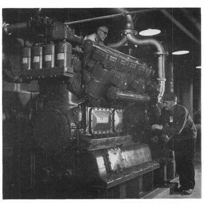
AUXILIARY DIESEL equipment in Sandia Lab Heating Plant is maintained by Joseph Wynn, top, and Salome Ramos, both 4514-2. In the event of power outage during the night, the men will put diesel equipment into operation to provide emergency power.
